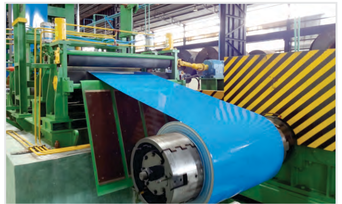
Galvanising/Pickling/Color Coating Line
